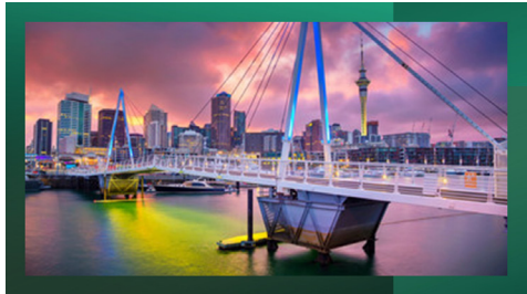
Auckland Walkway Bridges enable easy harbour access
